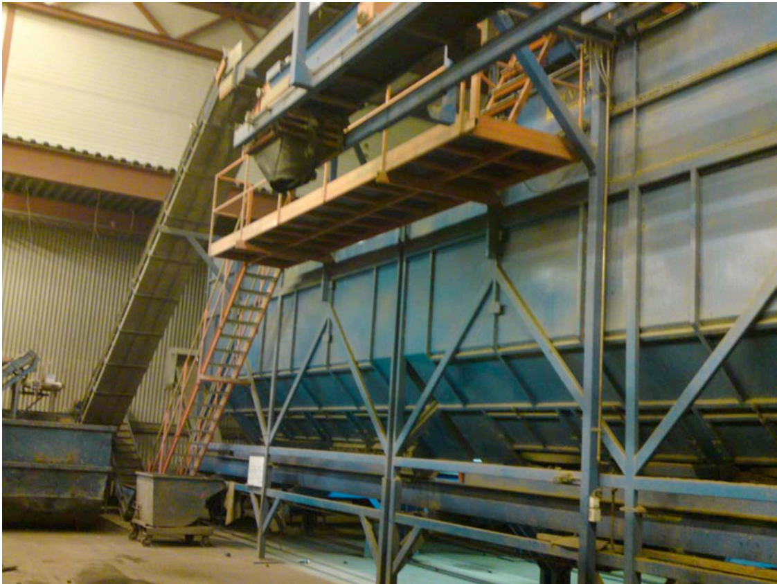
Steel hopper with a volume up 60 ton.
